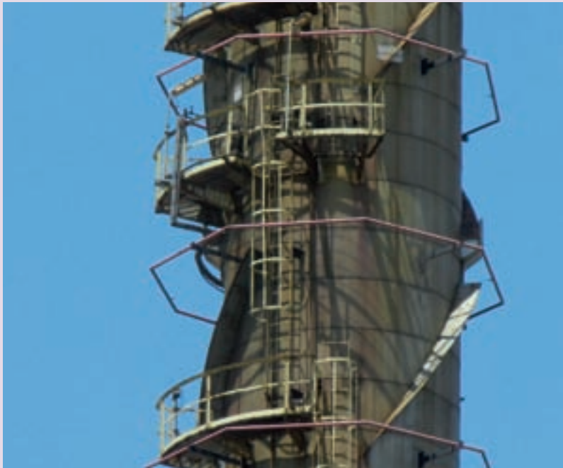
Figure 3: example of a poorly-designed and difficult-to-maintain deluge system installed on a process tower.
